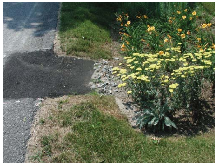
Shown at right: Bioswale to process stormwater run-off from the road.
