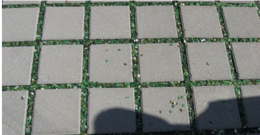
Paving blocks laid across a surface with spaces in between allow water to filter into the ground.
