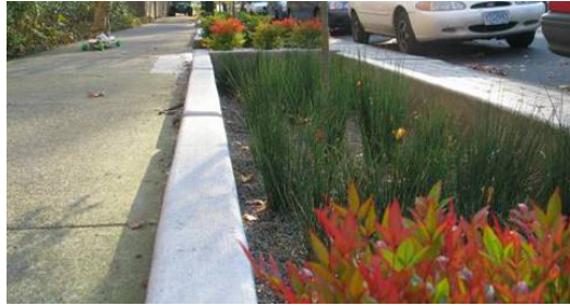
Stormwater planters are contained vegetated areas that collect and treat stormwater.
