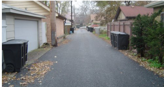
Permeable pavement allows rain and snow melt to infiltrate through, to be filtered into the ground.
