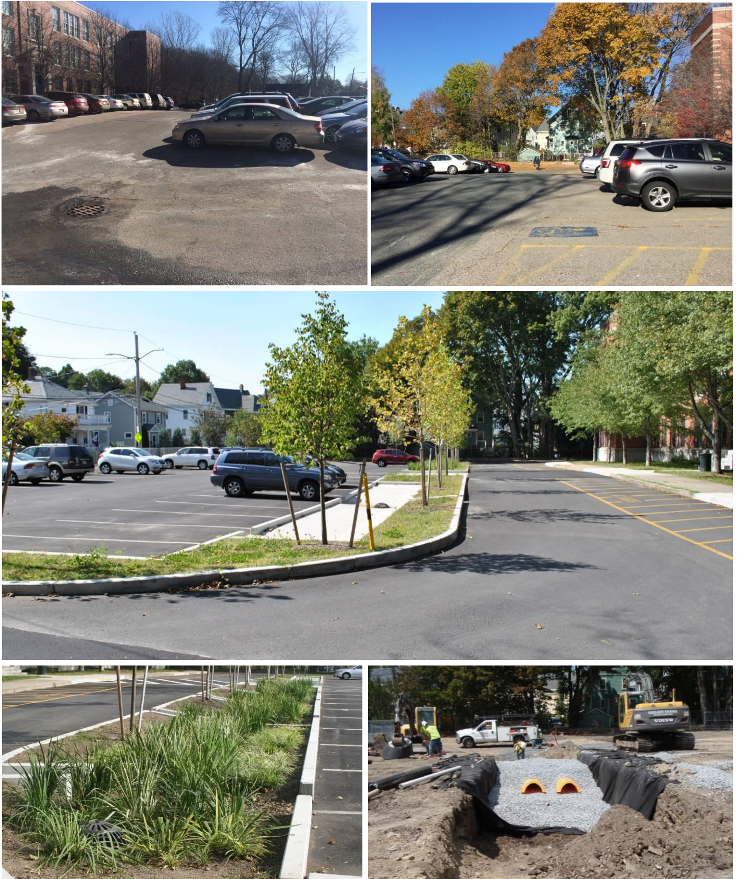
Figure 7. Before and after photos of bioswale and underground chambers in the rear parking lot.
