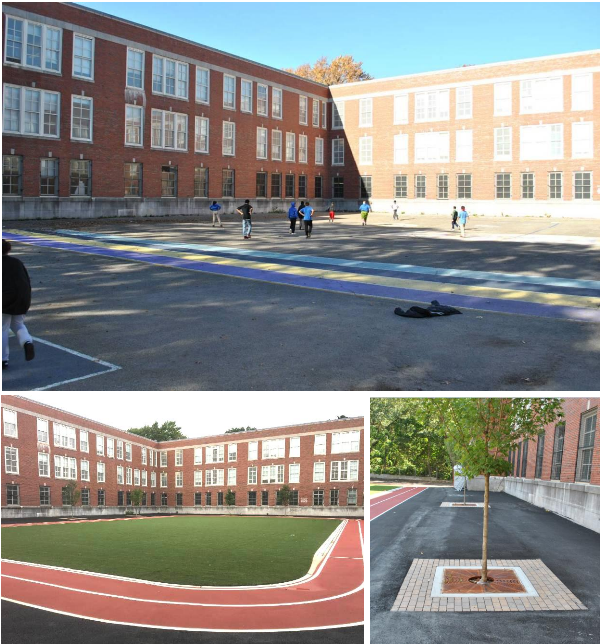
Figure 8. Before and after photos of the interior courtyard conversion to field with perimeter tree pits.
