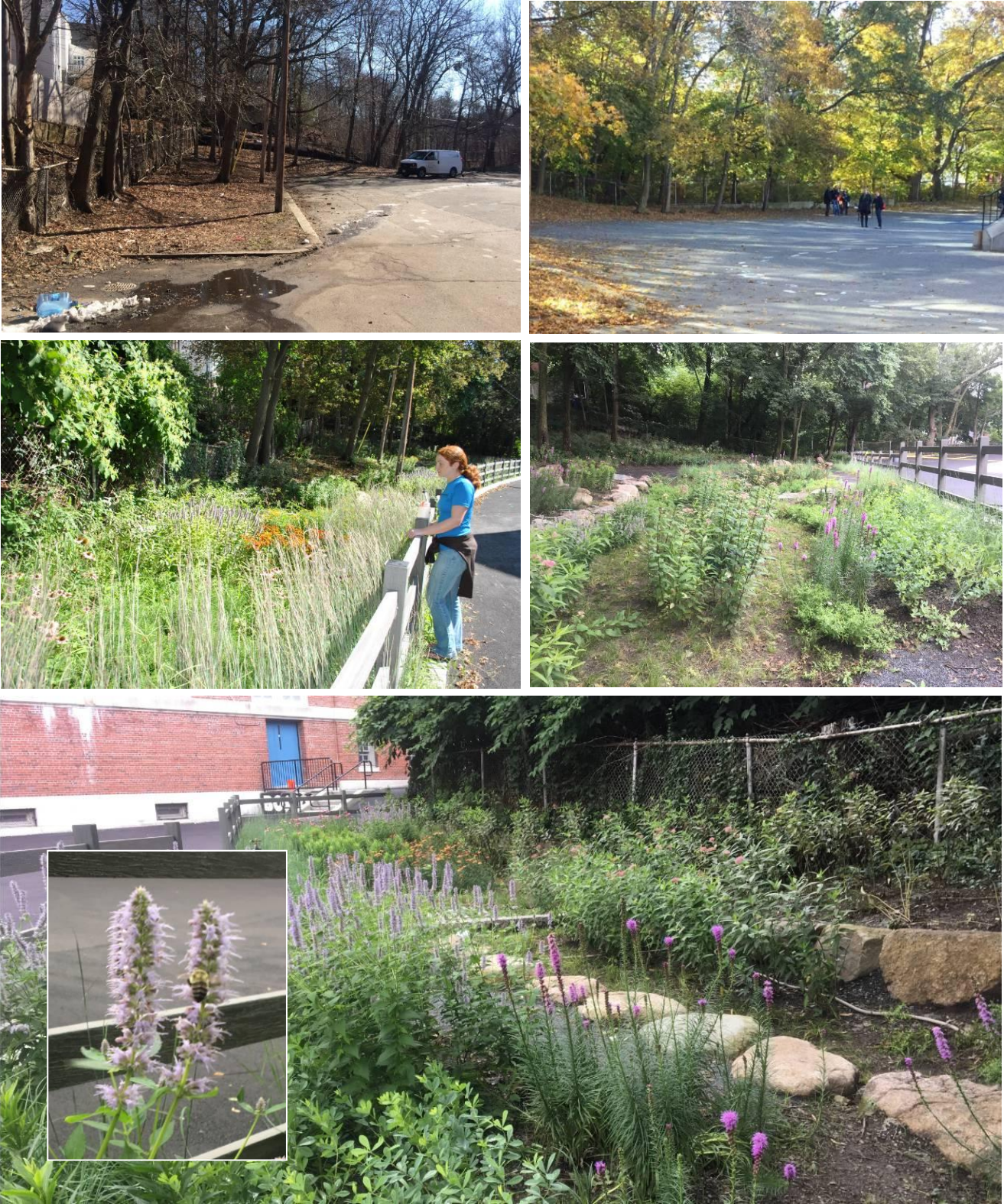
Figure 9. Before and after photos of the eastern corner conversion to bioretention.
