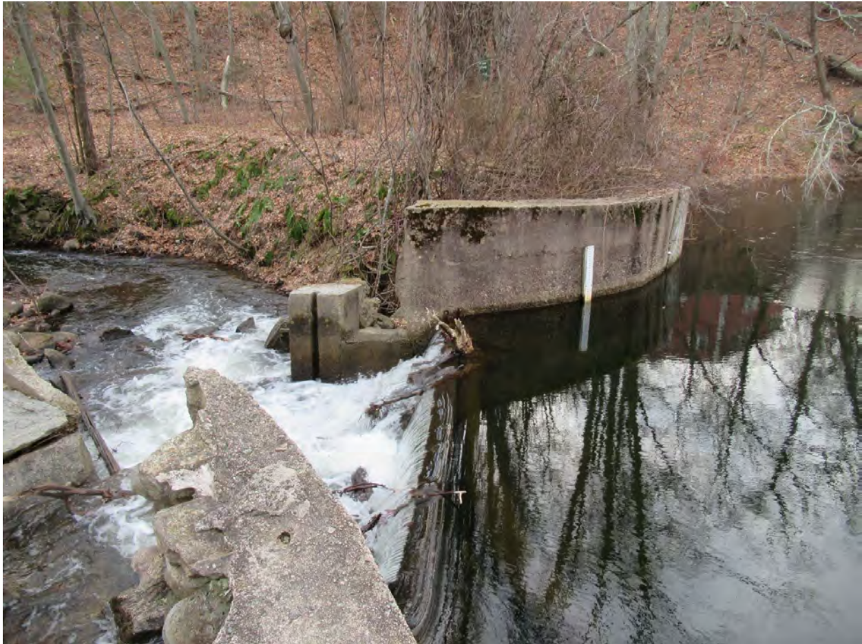
Figure 1. Spillway at Eagle Dam (Wrentham, Massachusetts)
