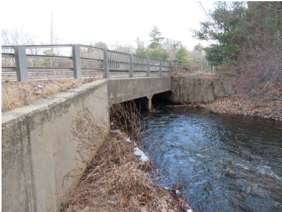
Photograph No.: 8 Route 140 crossing over Eagle Brook
