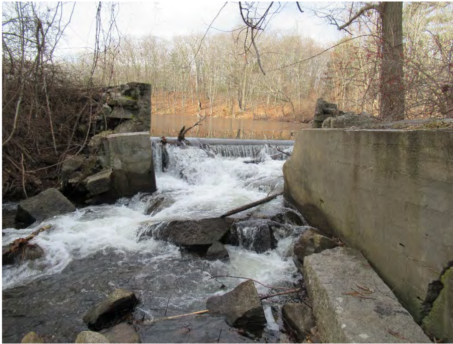
Photograph No.: 3 Downstream view of spillway-Eagle Dam
