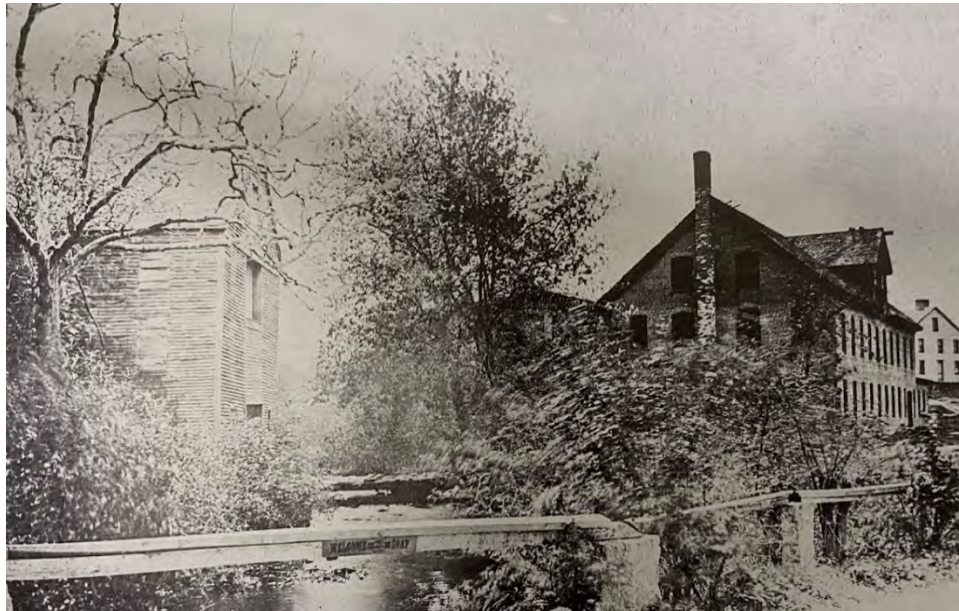
Figure 6. The Eagle Mill, also called the Eagle Manufacturing Company, was located between Franklin Street and Eagle Dam. All that remains is part of the rear foundation wall, now serving as a low retaining wall. The Whiting home can be seen at the right rear (source Wrentham Historical Commission).
