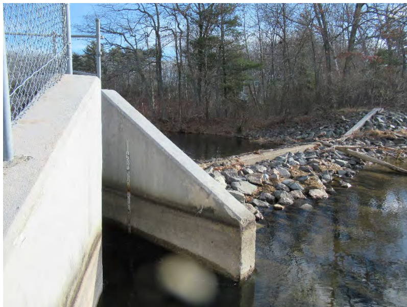
Photograph No.: 9 Red Dam spillway during drawdown
