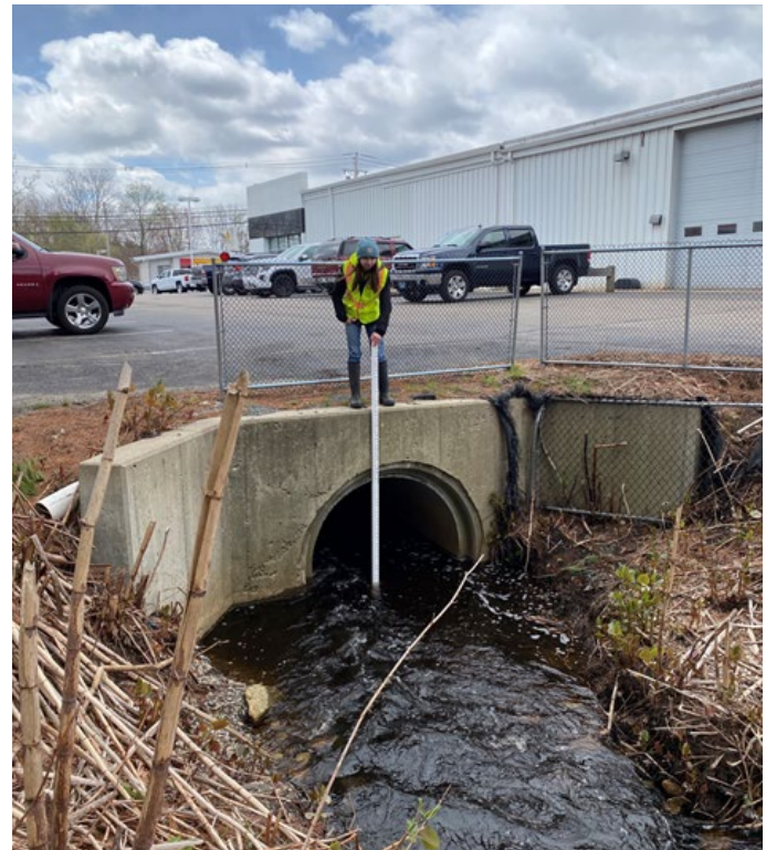
FIGURE 2.3 Photo showing a field team member measuring the diameter of a culvert.
