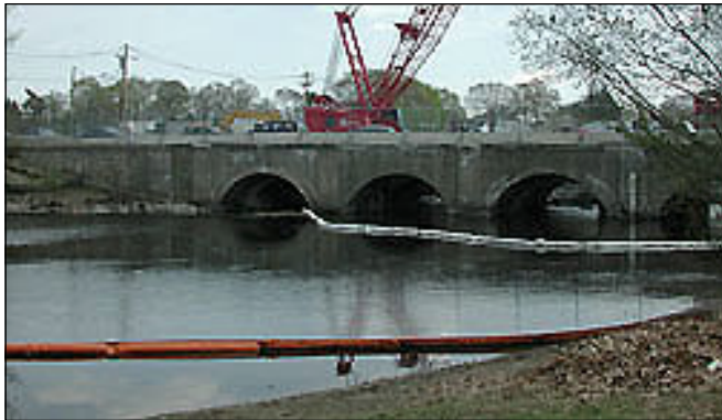
Construction equipment at Rte 109 leaked diesel oil.
