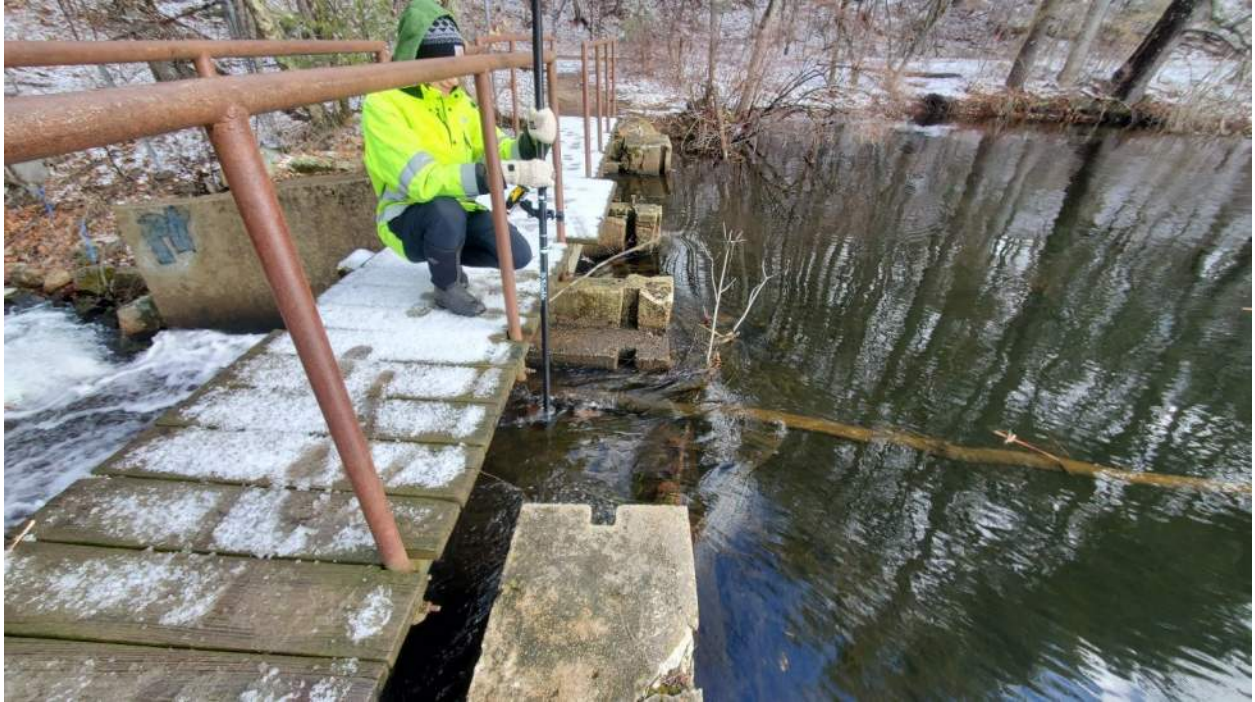
Photo 7: Bush Pond Dam (MA01158) looking at the spillways from the dam embankment. The spillways consisted of three stoplog-controlled channels.
