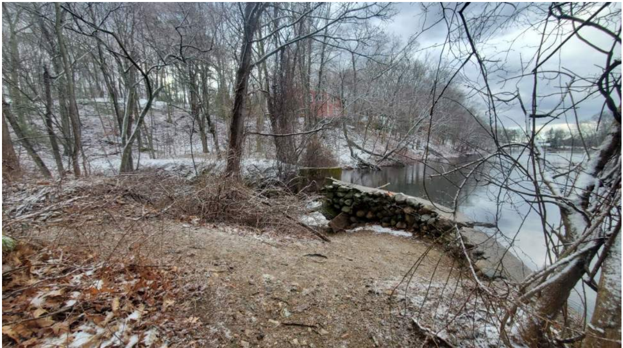
Photo 2: Eagle Lake Dam (MA02263) looking upstream at the primary spillway.
