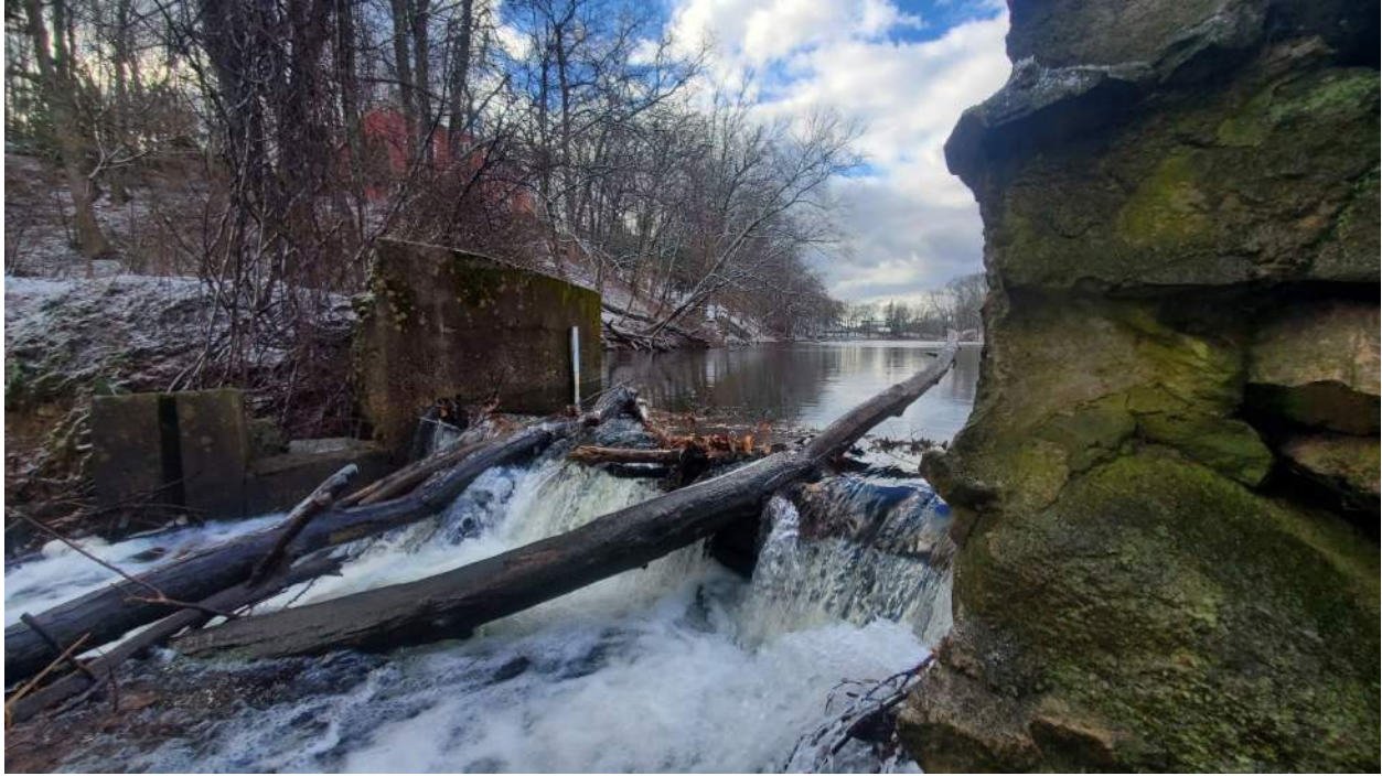
Photo 3: Eagle Lake Dam's (MA02263) primary spillway looking upstream. A staff gage is located on the right training wall.
