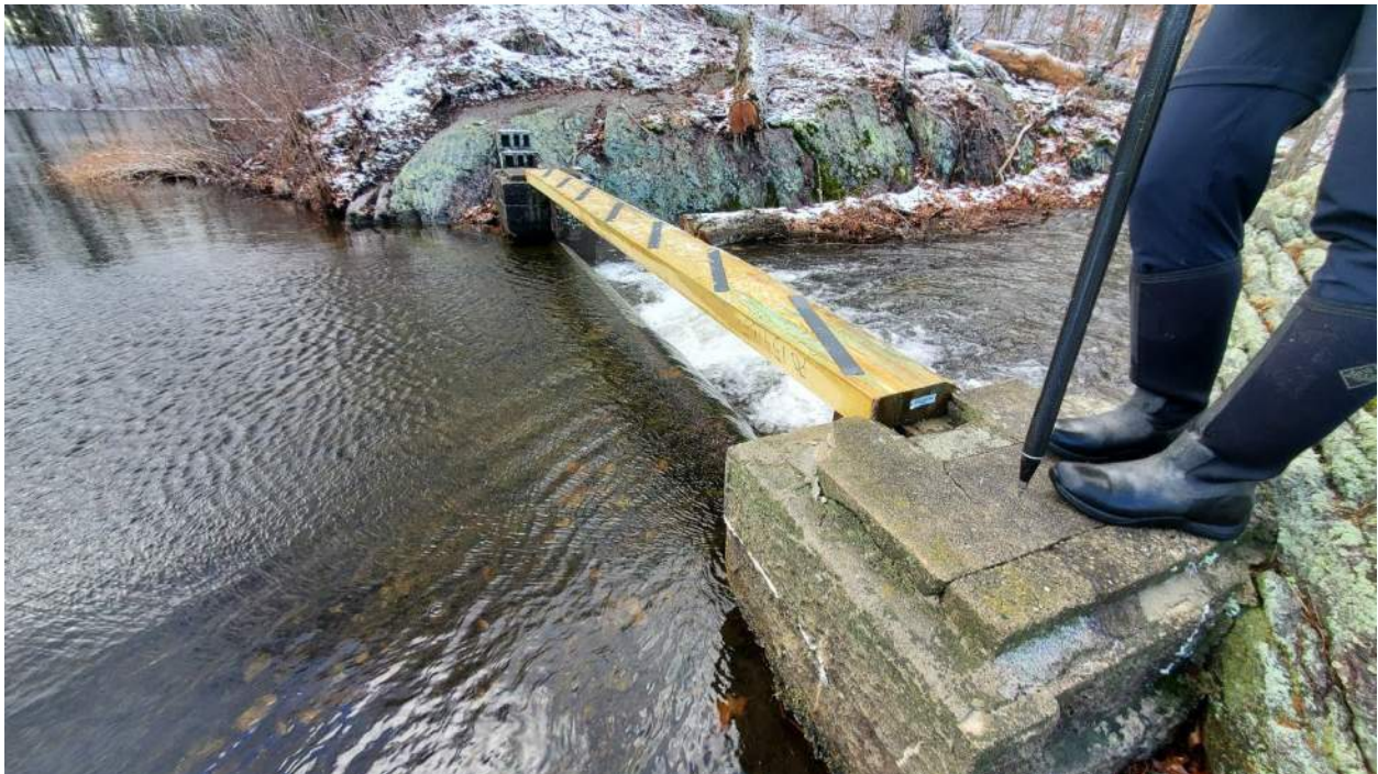
Photo 4: Unnamed dam at Mill Pond primary spillway. The primary spillway appeared to be a broad crested weir with a fixed angle iron.
