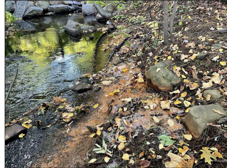
Photo No. 20.: Observed seepages with iron oxide flocculant approximately 15 feet downstream of the downstream channel left wall.
