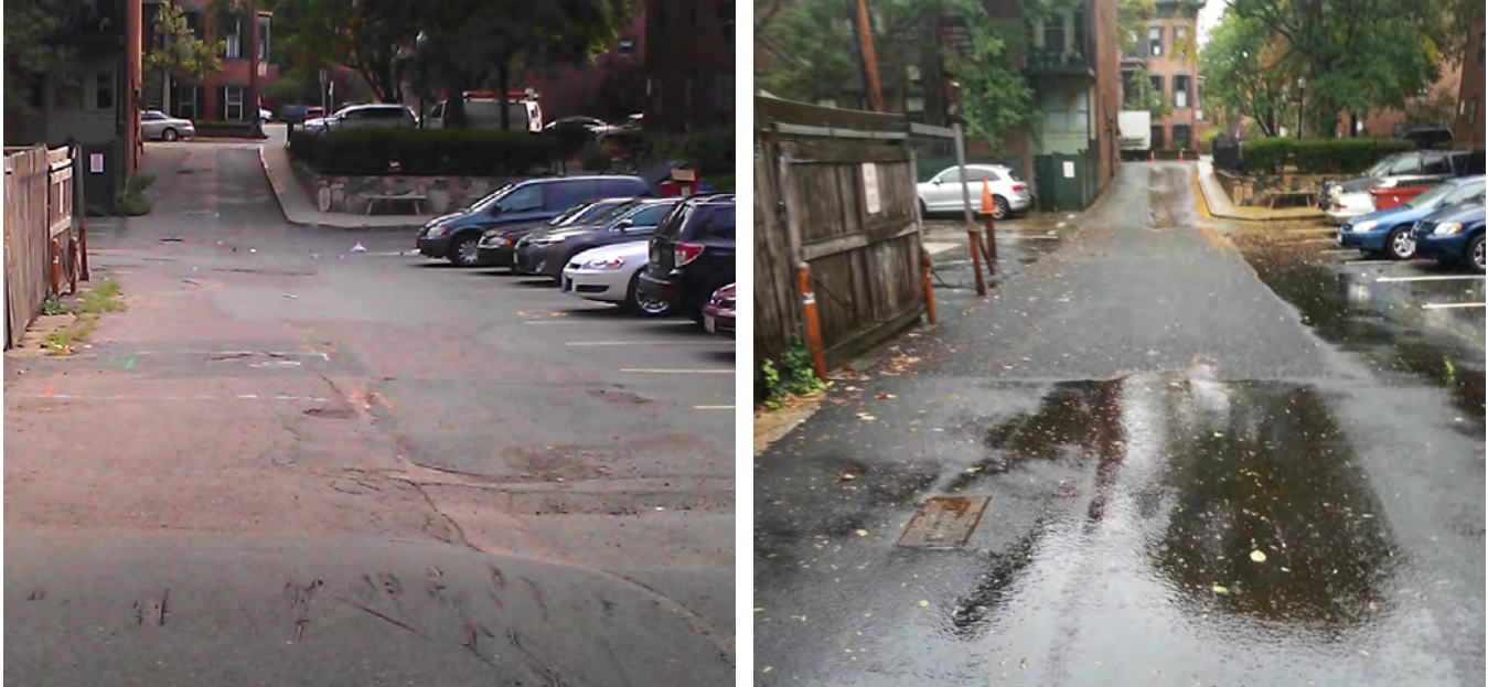
Figure F: Alley Before and After Construction
